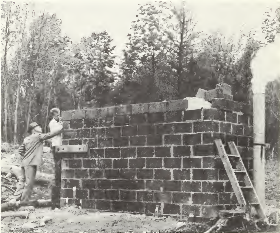
Figure 5.--Slabs and edgings can be used to make charcoal. Small kilns like this one have proved profitable in other parts of the Northeast.
